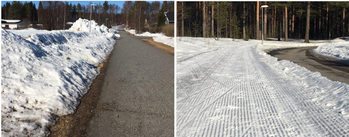
Figure 21. Example of a simple utilisation of snow to deliver recreational ES. Left: a swale used for snow storage only. Right: a swale is used as skiing track during winter. Both pictures taken in April in Luleå, northern Sweden.
