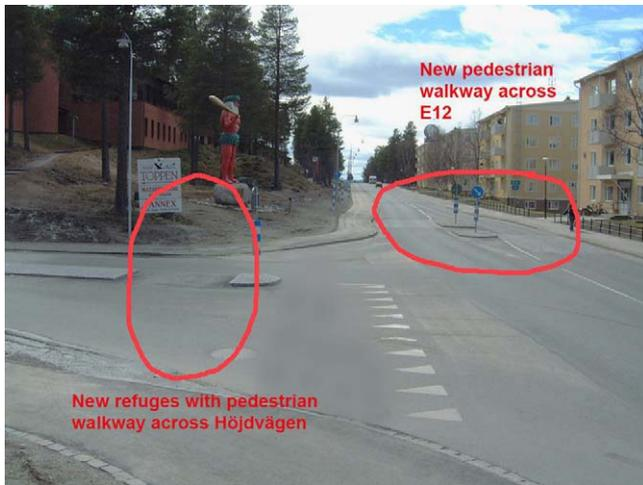
Fig. 2. Intersection Höjdvägen—E12 after reconstruction with a pedestrian walkway. View southwards along the E12.
