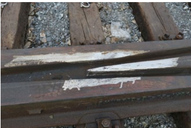
Figure 5. Artificial introduced realistic wear on crossing as input to AI.
