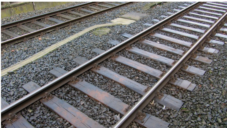
Figure 4.: Railway with wooden sleepers (source Wikipedia)
